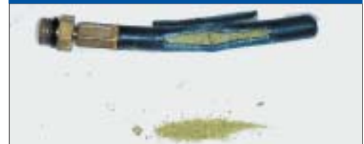
When this service hose from a recovery/recycling machine was cut open, it was found plugged with hardened sealer material.
